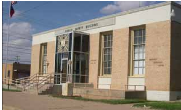
Illustration 11-2 Public Safety Building
