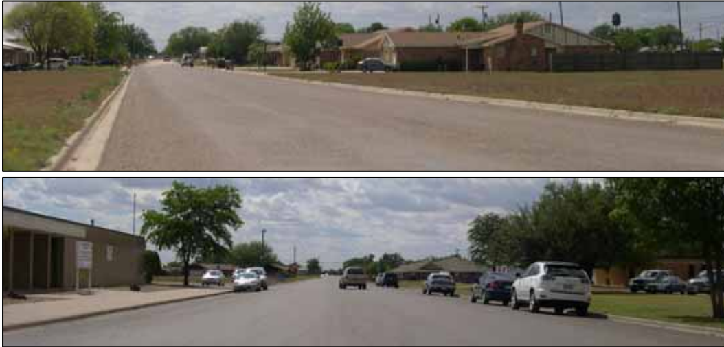
Illustration 10-4 Examples of Streets in Brownfield that Accommodate Storm Water via Surface Drainage and do not use Storm Sewers.
